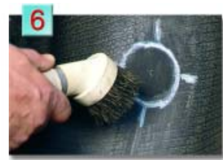
6. Remove buffing dust with a vacuum, then clean the buffed area with cleaner fluid and a scraper to avoid contaminating the injury channel.
