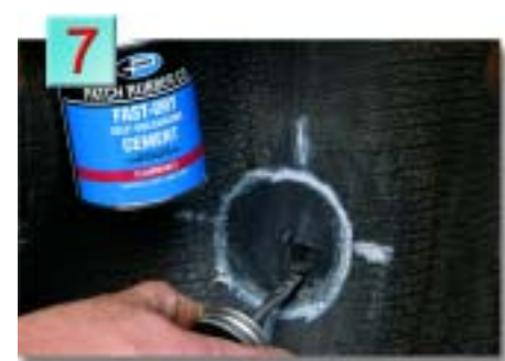
7. Apply an even coat of Patch Rubber Fast-Dry Self-Vulcanizing Cement to the buffed area. Allow to dry completely. Drying time will vary depending on temperature and humidity.
